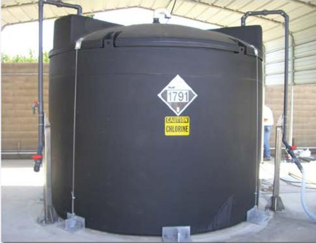
**SAFE-Tank® Double Wall Tank System**
