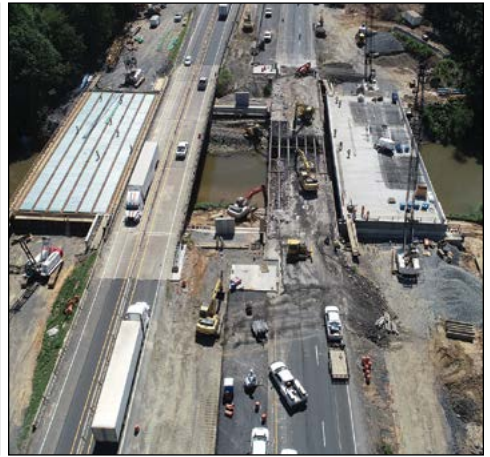
ARKANSAS PROJECTS. Top photo, Michael Baker did design work for the widening of Highway 70 from Benton to Hot Springs. Above left is the Maumelle interchange. Above right is the DeRoche Creek lateral bridge slides project – the first of its kind in Arkansas.
