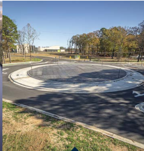
Location: Little Rock, Arkansas Mabelvale Pike Roundabout
