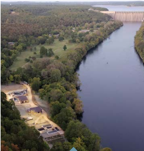
Location: Bull Shoals, Arkansas Bull Shoals Water Treatment Plant
