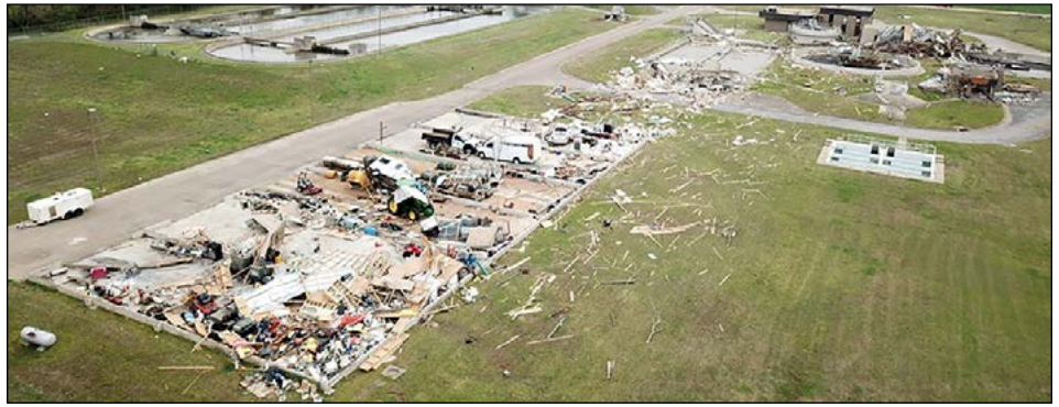
TOTAL DESTRUCTION. Not much was left of the wastewater facility. It will be replaced with a new one costing $18 to $20 million. Photo courtesy of Crist Engineers.
