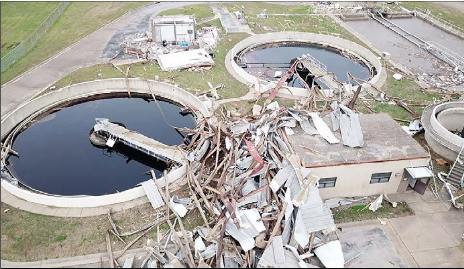
TORNADO AFTERMATH. The tornado that struck Wynne destroyed the town’s wastewater treatment facility. To keep sewage from backing up into homes and covering the ground at the plant, General Manager Blake Marotti diverted the wastewater to an equalization basin. It became part of the midterm response. Photo courtesy of Crist Engineers.
