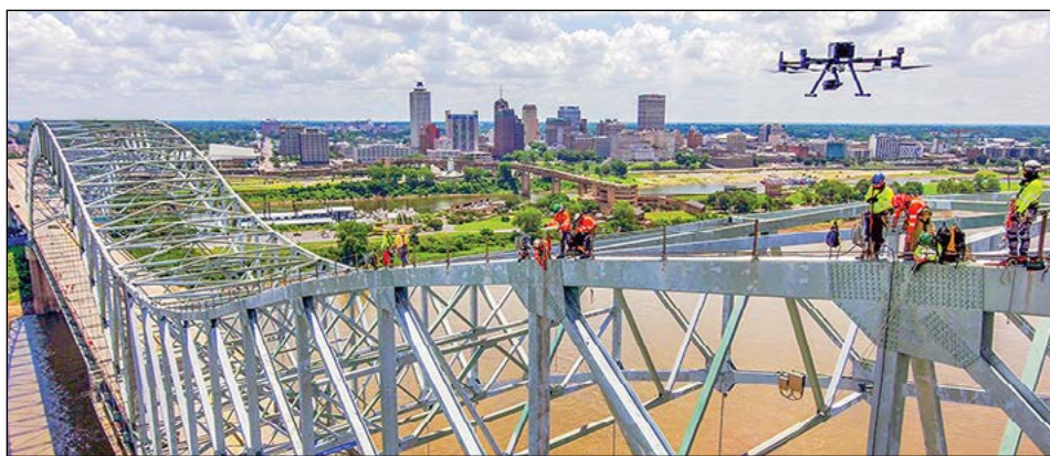
MICHAEL BAKER INTERNATIONAL engineers inspect the Hernando de Soto Mississippi River bridge using unmanned aerial system technology and rope access techniques.
