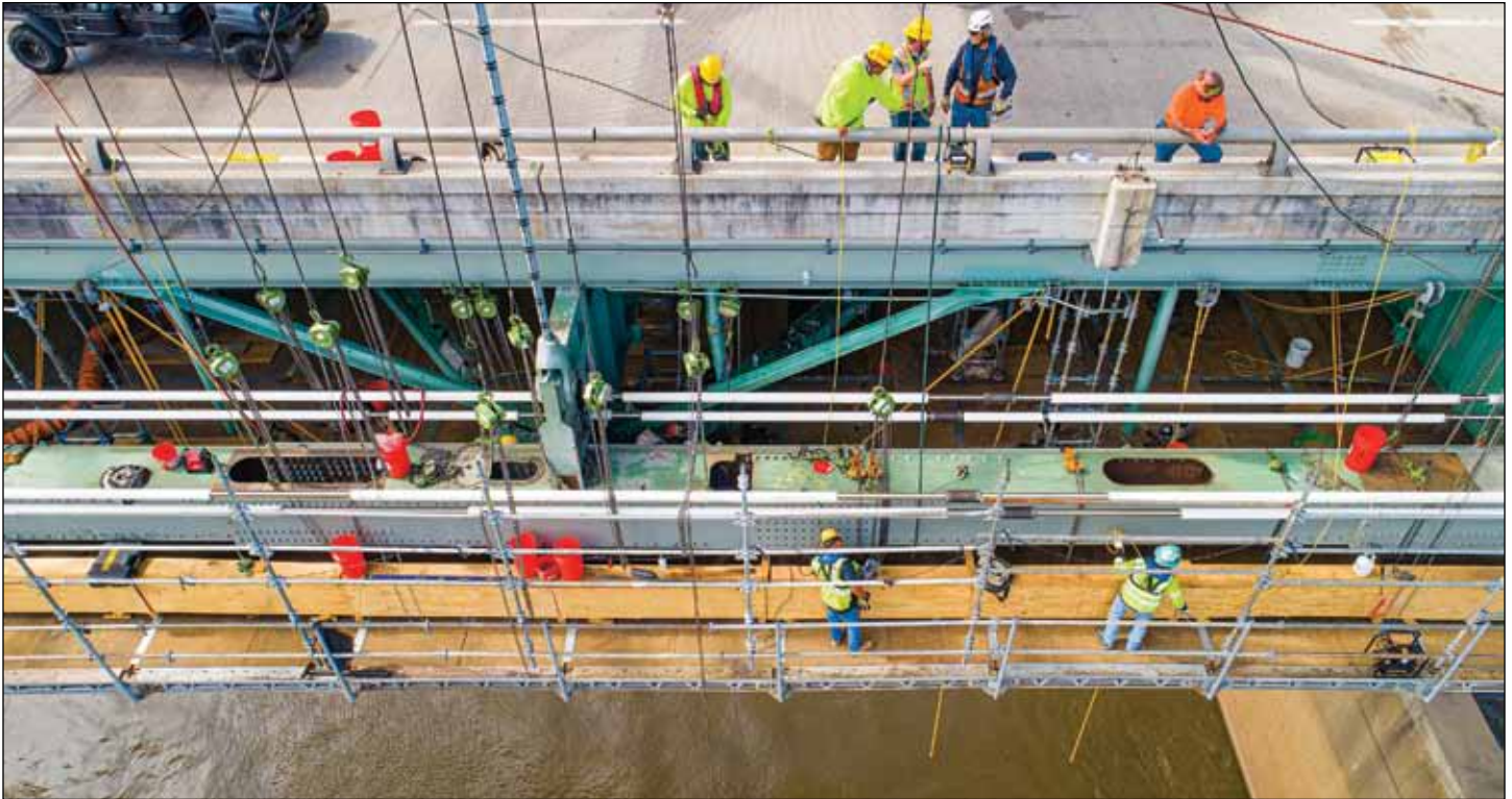
WORKERS make repairs to the Hernando de Soto Bridge, which has been closed since May 11 after Michael Baker International inspectors discovered a significant fracture in one of the bridge's two supporting tie girders.
