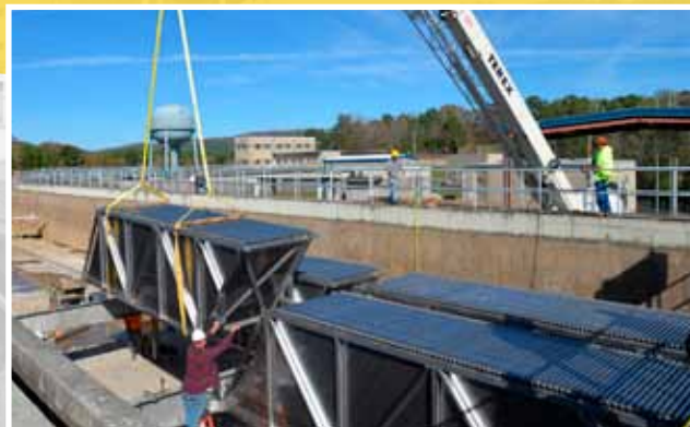
Plate Settler Installation - Hot Springs Water Utilities
