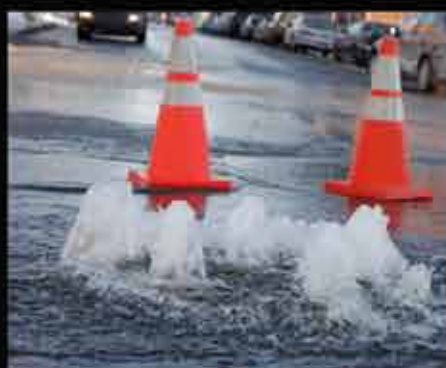
Surcharging can result in sanitary sewer overflows
