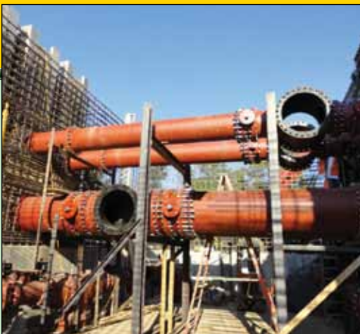
Filter Gallery Piping Clarksville Light & Water Company
