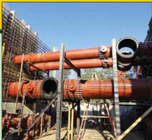
Filter Gallery Piping Clarksville Light & Water Company
