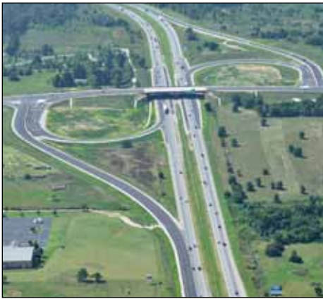
BUSY SPRINGDALE. The interchange relieves congestion and was opened months ahead of schedule.
