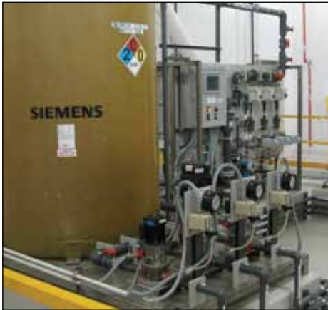
A CHLORIDE DIOXIDE GENERATOR at one of Central Arkansas Water's plants is pictured. Photo courtesy of Central Arkansas Water.
